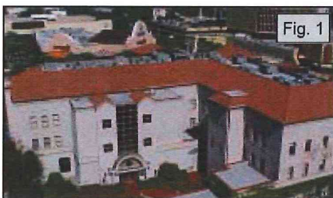
Figure 10: Examples of appropriately placed utilities i.e. located on the roof & screened by parapet walls, with both aerial & ground views.
